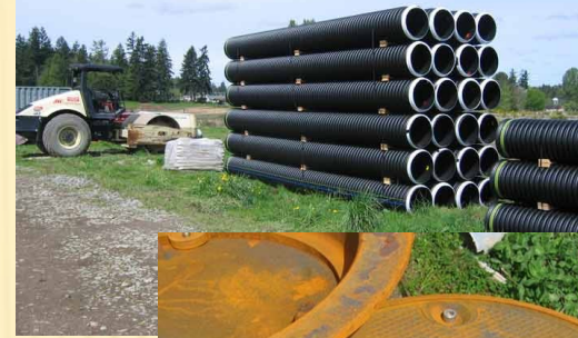
Step 5. Bring in lots of drain pipe
